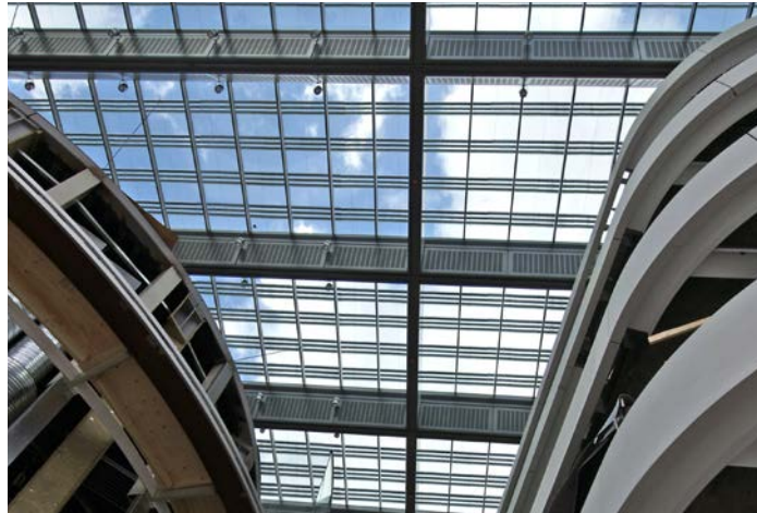
Figure 9 - Danish Television in Ørestad with photovoltaic on the roof
