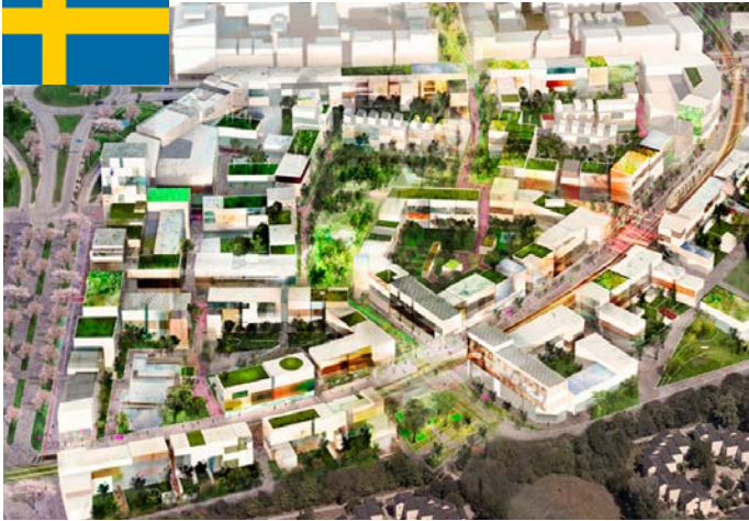
Figure 3 - First stage of development. (Source: © Atkins)
