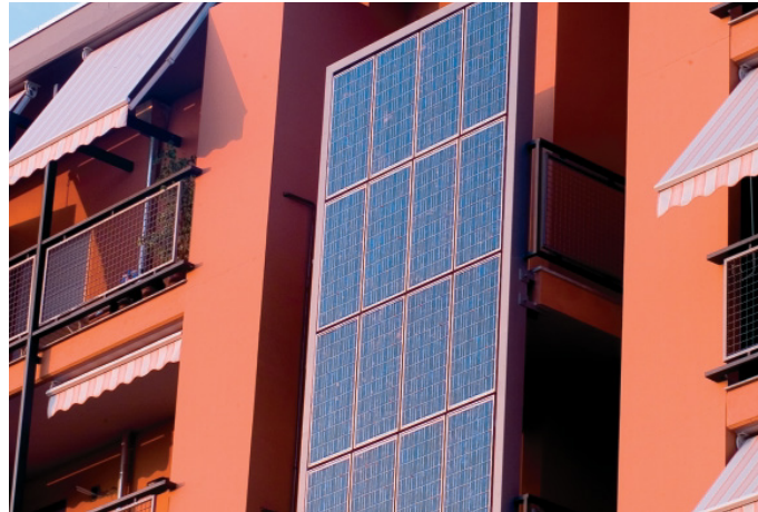
Figure 8- System modular pattern [3] The PV panels installed on façade of the row houses of the district (Source: © PierFranco Robotti).
