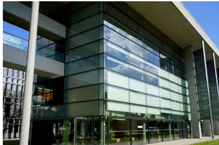
Figure 15 - Centre of Biotechnology and the Environment. (Photo: © Margarethe Korolkow)
