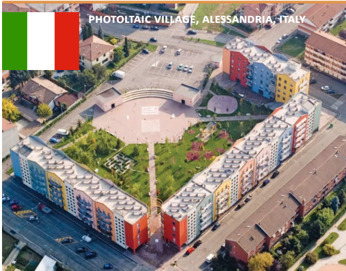
Figure 3 - Aerial view of the eastern area of the Photovoltaic Village. (Source: © Municipality of Alessandria)
