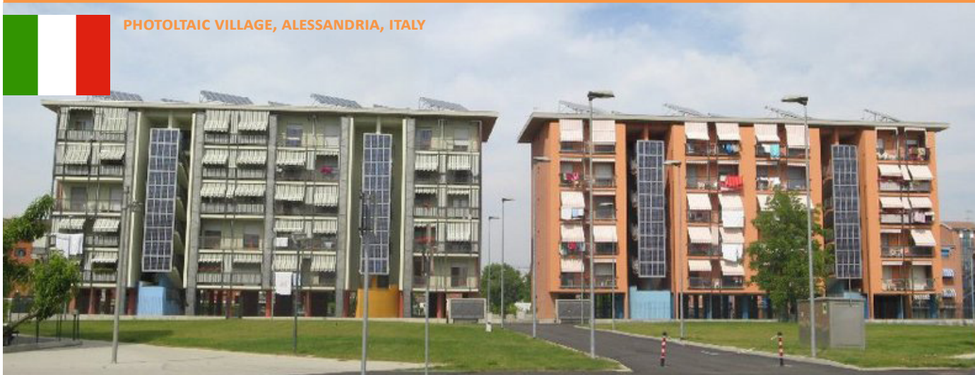
Figure 5 - PV panels installed on façade of the row houses of the district. (Source: © Google)
