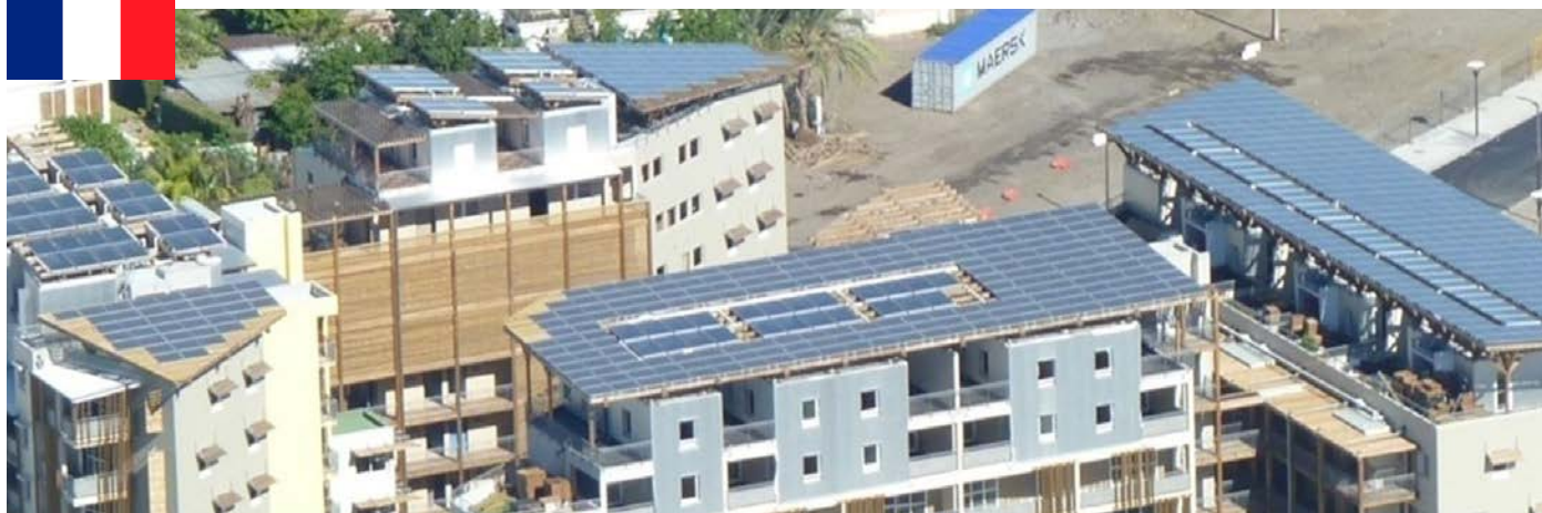
Figure 5 - Overview of the combined PV and solar thermal panels roof plant. (Source: © AP Architectures/ZAPMR)
