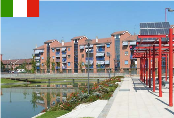
Figure 7 - Public green areas between the buildings and shelters with PV panels. (Source: © Municipality of Alessandria).
