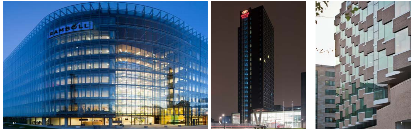
Figure 5 - Office building (a), Hotel (b) and school (c) - examples of buildings in Ørestad with photovoltaic
