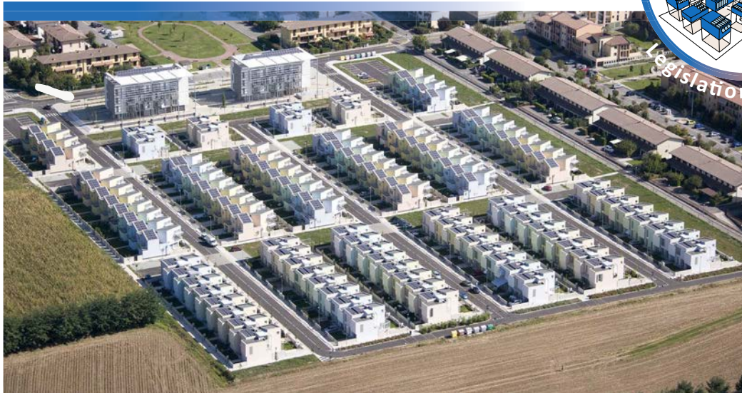
Figure 2 - View of the Violino district in Brescia, Italy. (Photo: © BAMSpoto - Basilio)
