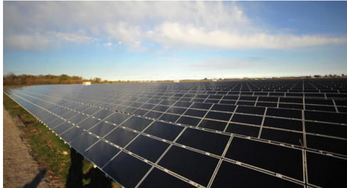
Figure 11 - Solar Panels. (Source: © Postmedia Network)
