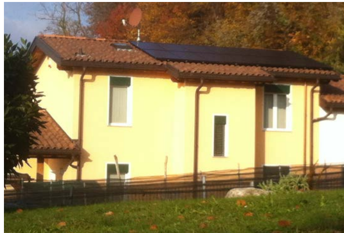
Figure 10 - New solar photovoltaic installation. (Photo/source: SUPSI)
